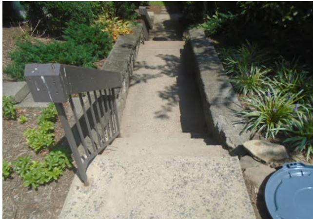
Retaining walls between 11630-11636 have slight leans to them. Walls are structurally sound at this time but should be monitored and repaired when needed.
