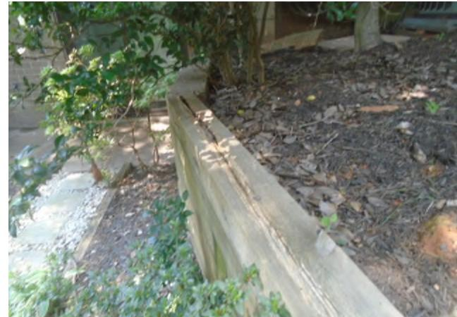
Top member of wood retaining wall is deteriorating. Member can be replaced without replacing the entire wall. When total replacement is needed, install a low maintenance modular block system.
